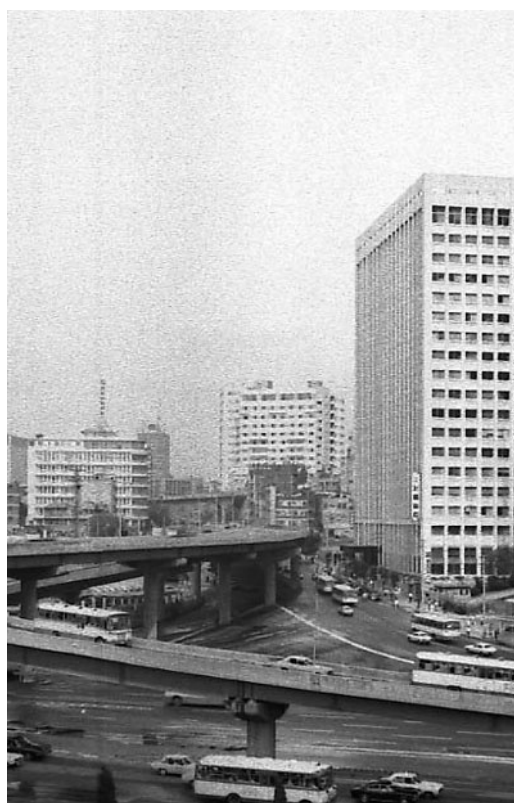
The whole view of the Seoul Station Overpass with the Mallijae-Toegy-ro section under construction in 1975. Credit: Seoul Metropolitan Government
